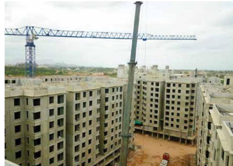
Construction in prefabricated concrete elements combines unrivalled speed of progress in construction with safety at work and consistency in the high quality of the precast concrete elements. To date 27,169 solid walls and slabs have been constructed for 1,008 residential units at Brigade Orchards. On average, a further 50 residential units are completed each month.
