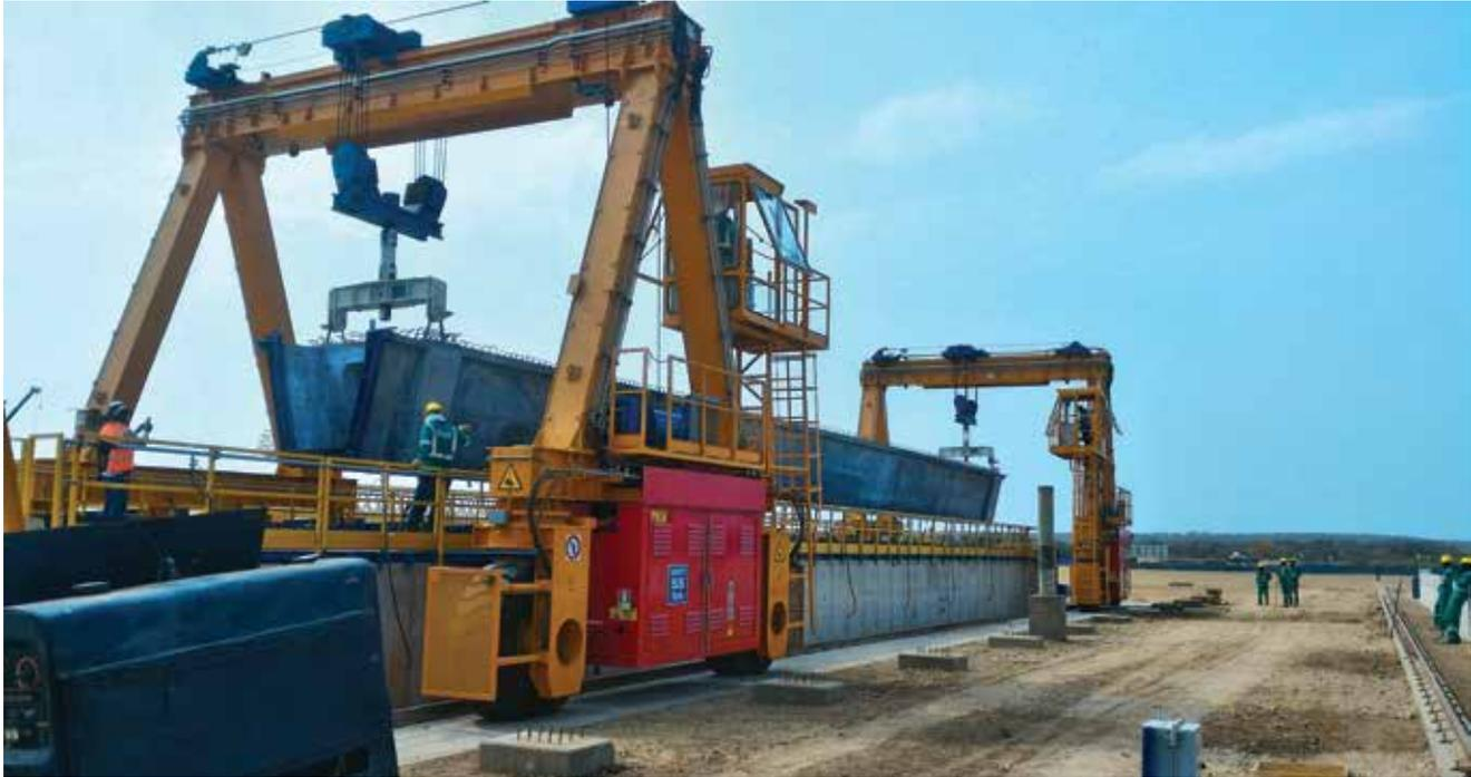
Two gantry cranes load a total of 387 concrete elements on to special HGVs, which transport them to the construction site.
